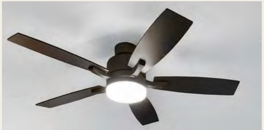
Black 5 Blade Ceiling Fan Installed
